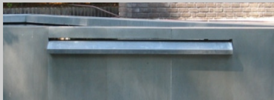
Two connected ponds in zinc, with a natural height difference of 110cm
