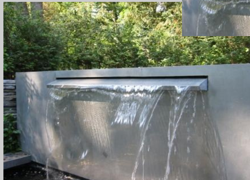
Two connected ponds in zinc, with a natural height difference of 110cm
